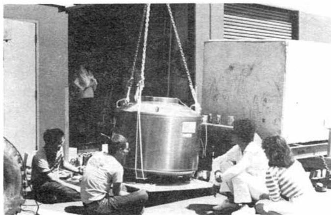
Mounting the A-2542 dewar on its plywood base.
