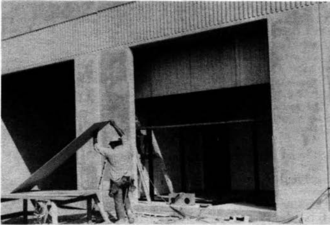
Office construction at the new facility
