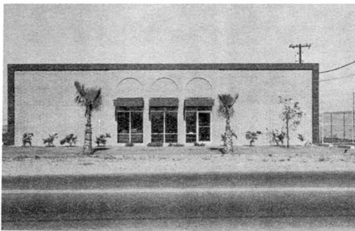
Cryocare manufacturing facility owned by Mr. Hope. Never fully used.
