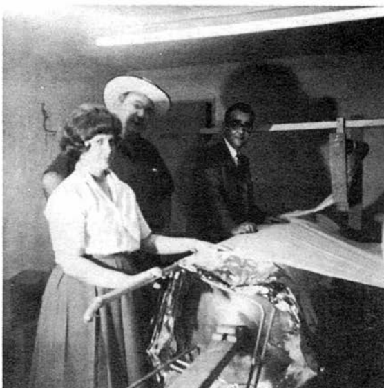
Barbara Kraver and Ed Hope (with hat) wrapping glass matt and aluminum foil on inner vessel of first cryocapsule.
