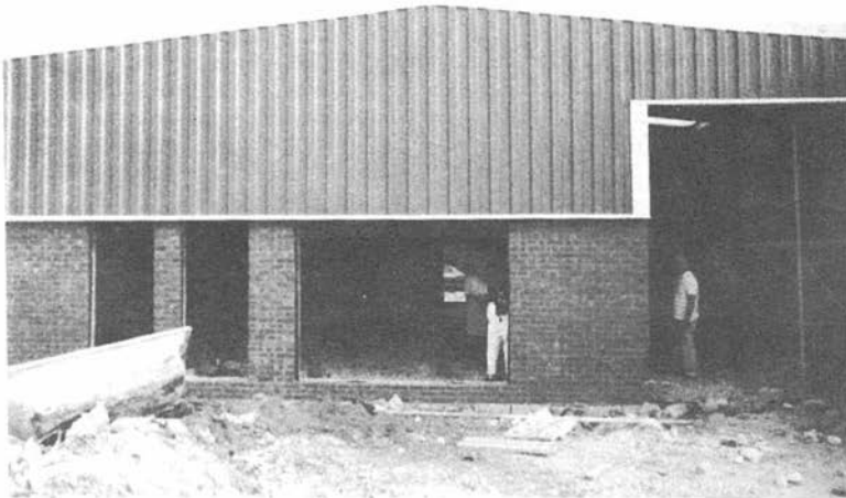
External view of English facility now being constructed
